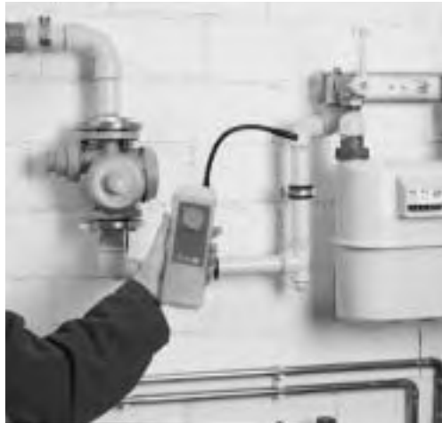
Fig. 26: Detecting leaks in gas pipes using testo 316
